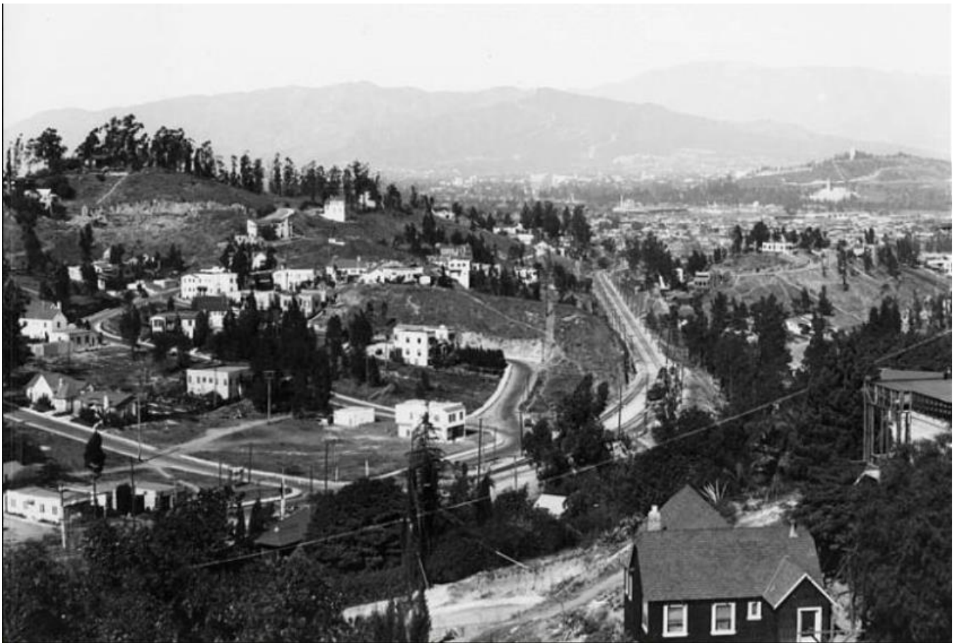
Figure 6-1. Pacific Electric Edendale Cut, 1930 [Wikimapia; Metro Library and Archive for date of 1930]
